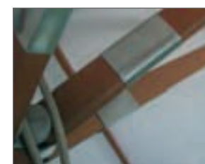
FASCETTE METALLICHE SULLE STECCHE WRAPS ON THE RIBS
